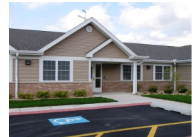
Sterling Apartments 2104 East 23rd St. Sterling, IL 61081
