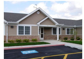
Sterling Apartments 2104 East 23rd St. Sterling, IL 61081
