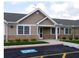
Sterling Apartments 2104 East 23rd St. Sterling, IL 61081
