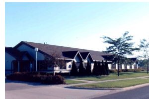
Fairview Apartments 555 Fairview Drive Rochelle, IL 61068
