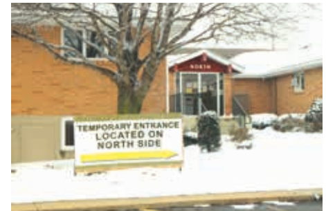
Sinnissippi Centers' Dixon office has a temporary entrance during construction on the side that faces Illinois Route 2.
