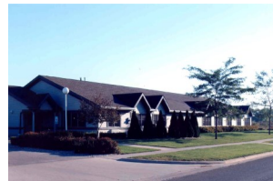
Fairview Apartments 555 Fairview Drive Rochelle, IL 61068
