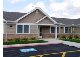
Sterling Apartments 2104 East 23rd St. Sterling, IL 61081
