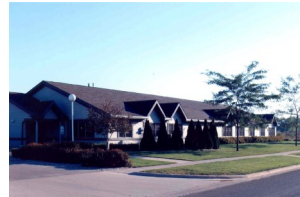
Fairview Apartments 555 Fairview Drive Rochelle, IL 61068
